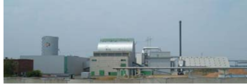
This power plant in Denmark uses the waste heat to heat green houses nearby.
